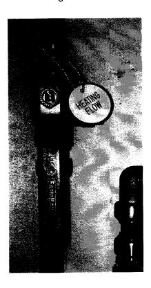
The heating system is furnished with 2 No. isolation levers which isolate the LPHW supplies to your manifold. The isolation valves are located in the services cupboard and are provided with a "HEATING FLOW" and a "HEATING RETURN" tag identifying the valves.
