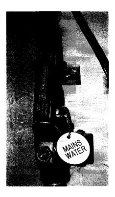
Your supply is furnished with a main isolation lever which isolates cold water supplies to your bath, wash hand basin, toilet, kitchen sink and other water utilising appliances. The isolation valve is located in the services cupboard and is provided with a "MAINS WATER" tag identifying the valve.
