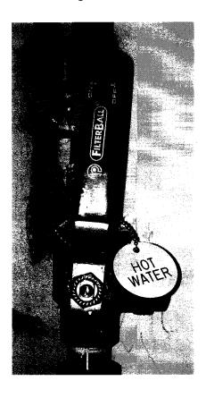
Your supply is furnished with a main isolation lever which isolates hot water supplies to your bath, wash hand basin, kitchen sink and other water utilising appliances. The isolation valve is located in the services cupboard and is provided with a "HOT WATER" tag identifying the valve.
