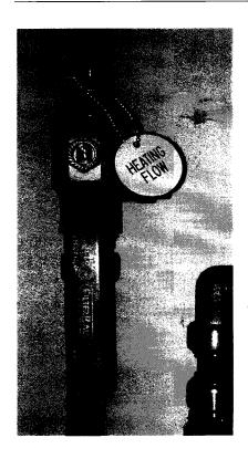
The heating system is furnished with 2 No. isolation levers which isolate the LPHW supplies to your manifold. The isolation valves are located in the services cupboard and are provided with a "HEATING FLOW" and a "HEATING RETURN" tag identifying the valves.
